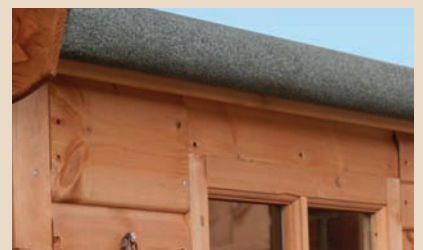
Rounded roof edges give a softer look and makes the roofing felt last longer.
