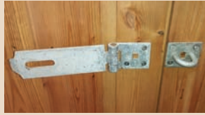
Heavy duty hot spelter galvanised fittings used on both shiplap cladding.
