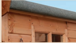
Rounded roof edges give a softer look and makes the roofing felt last longer.
