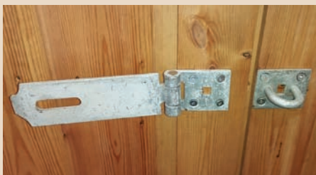
Heavy duty hot spelter galvanised fittings used on both shiplap cladding.
