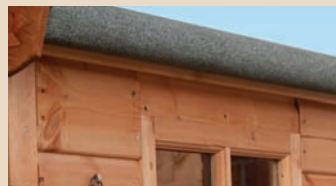
Rounded roof edges give a softer look and makes the roofing felt last longer.
